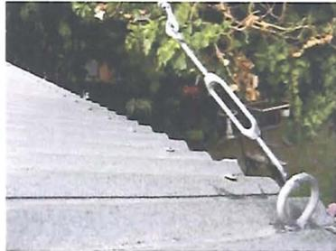
Turnbuckle ready to be tightened, but not for the last time..
